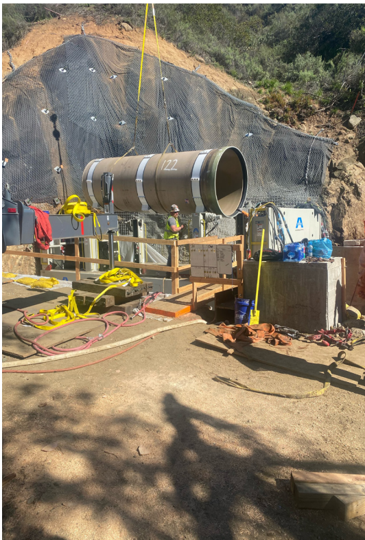
Tunnel liner being lowered. Oat Hills tunnel rehabilitation.
