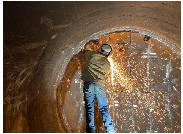
Pipeline 5 Reline bulkhead installation.
