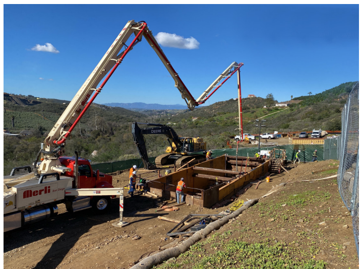
Closing access portal on Pipeline 5 Relining project 2023.
